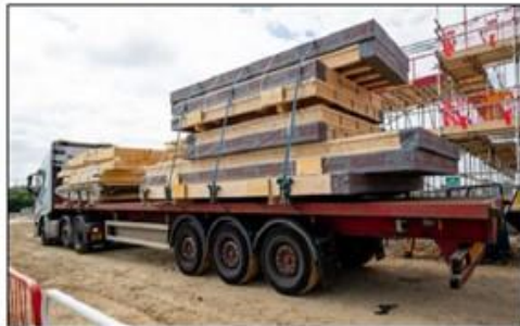
7 – Delivery to site
