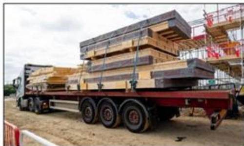
7 – Delivery to site
