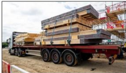
7 – Delivery to site
